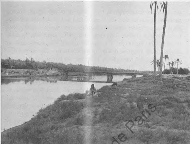
Jarbuiyah Bridge, looking down-stream.
