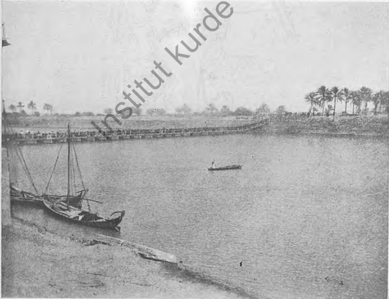
Bridge at Tuwairij from right bank.
