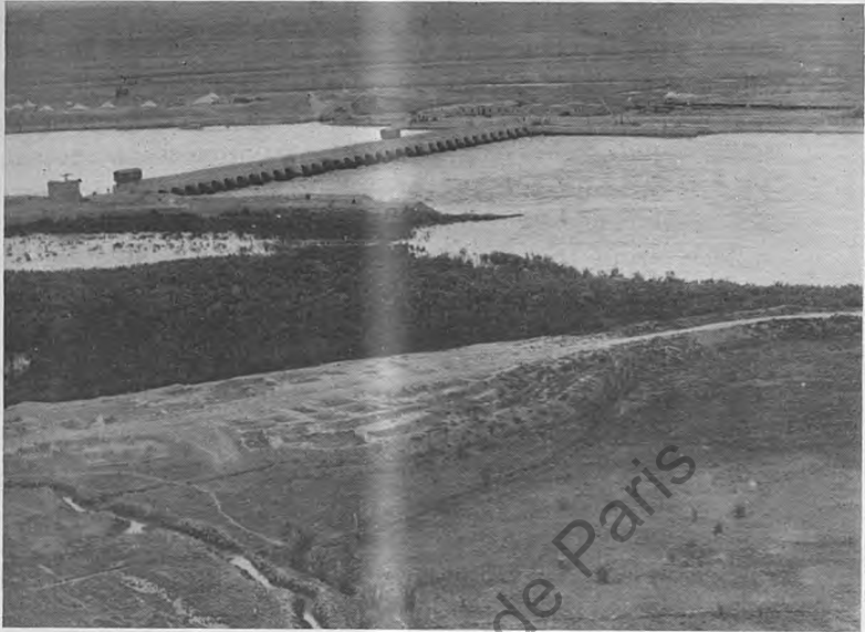
Hindiyah barrage from the west.
