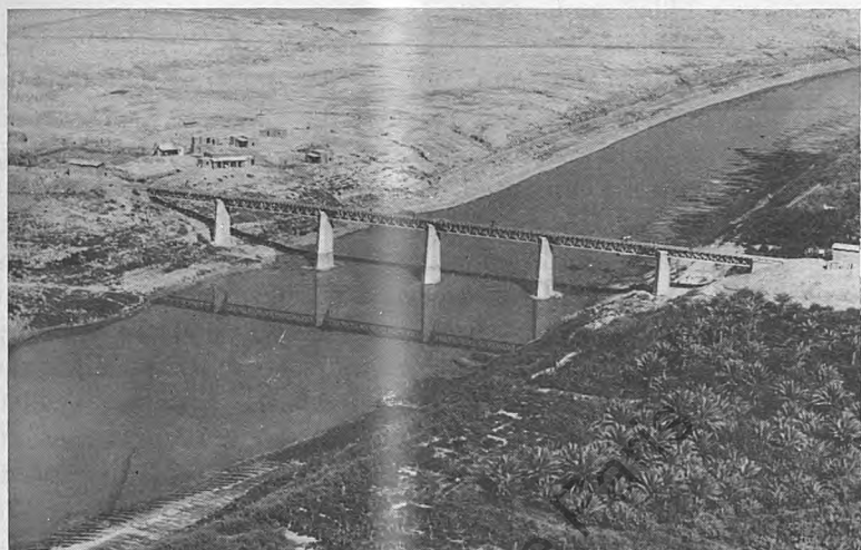
Bridge over Diyalah river near Baqubah.
