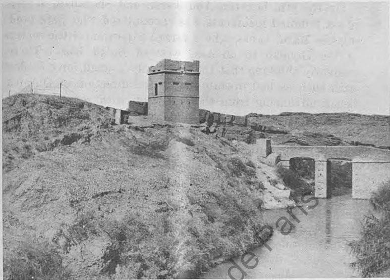
Blockhouse and regulator of Ruz Canal.
