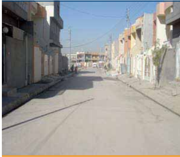
Figure 10.4 Badawa after Completion of Rehabilitation Works
