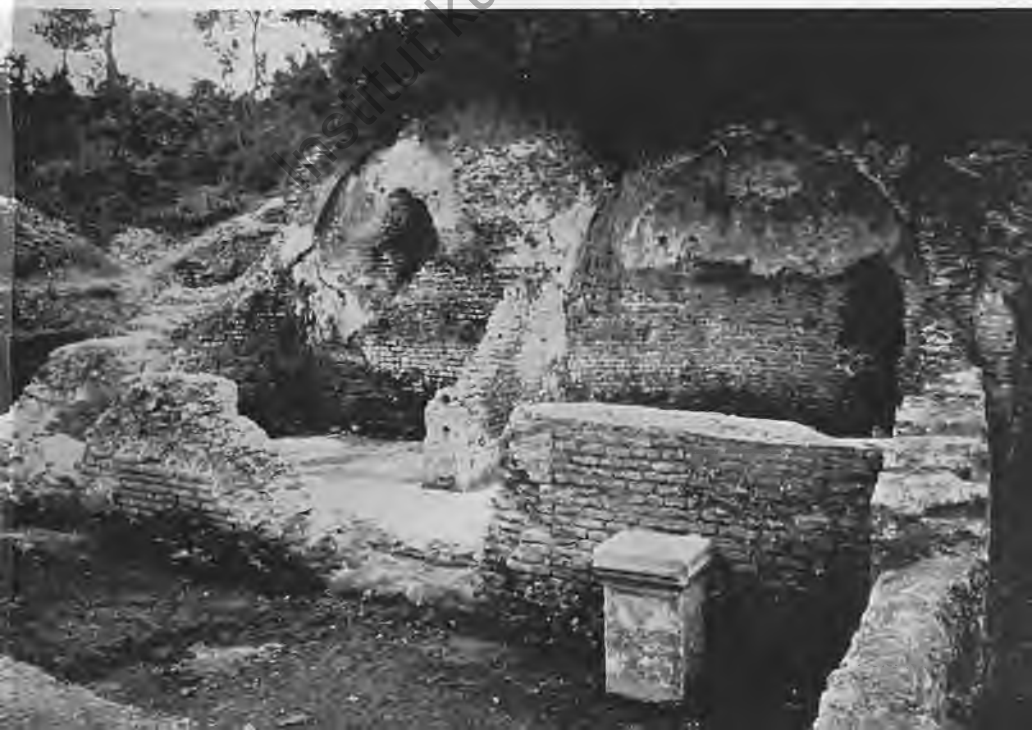
The bath buildings at Teano.
