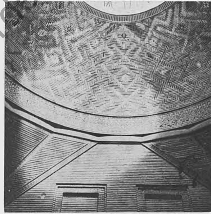
Res. 20 — Konya, İnce Minareli Medrese, kubbe.
