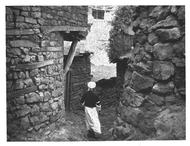
Fig. 16. Stone wall with inserted horizontal beams. Tawella.
