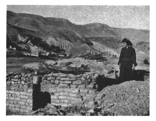
Fig. 19. Wall of mud bricks. Topzawa.
