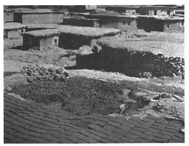
Fig. 18. Mud bricks laid out for drying on the hillside. Topzawa.
