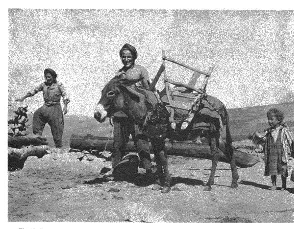
Fig. 17. Housebuilding. Clay and water are kneaded with the feet. Pebbles for foundation are transported by donkey. Topzawa.
