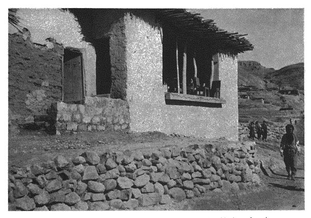
Fig. 20. Loggia with columns made of slim, barked poplar trunks with pieces of wood inserted as capitals. Topzawa.
