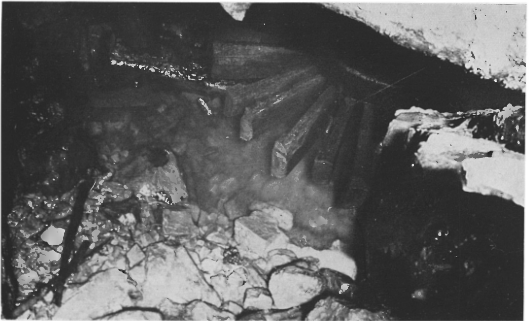
Plate 16. Turbine Water Mill. Rotor blades.
