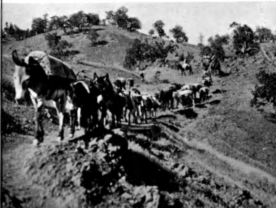
9. Mule Caravan transporting 'Juss' to Kani Rash (below)
