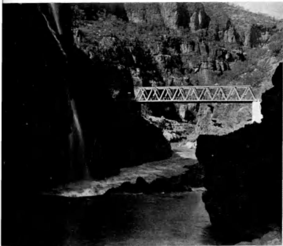
23. The Main Bridge over the Rowanduz River
